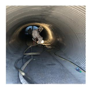
Superior Grouting Spray Liners utilizing Nukote Aegis \*, differ depending on the effluent type, abuse levels, abrasion, ground movement, substrate condition and other design variables. The application processes are similar, the liner formulation utilized is variable.
