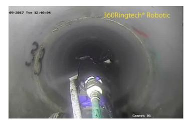
Liner formulations are interchangeable dependent on the effluent, providing versatility unmatched by conventional liners. The Nukote 360 Ringtech® robotic application process is identical, simply changing the elastomeric product utilized allows for use in all possible effluent types.
